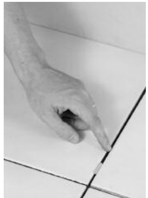
Method 3: Remove the grout 1/4" to 1/2" deep. Install sensor. Reinstall grout over the sensor and sensor wire.
